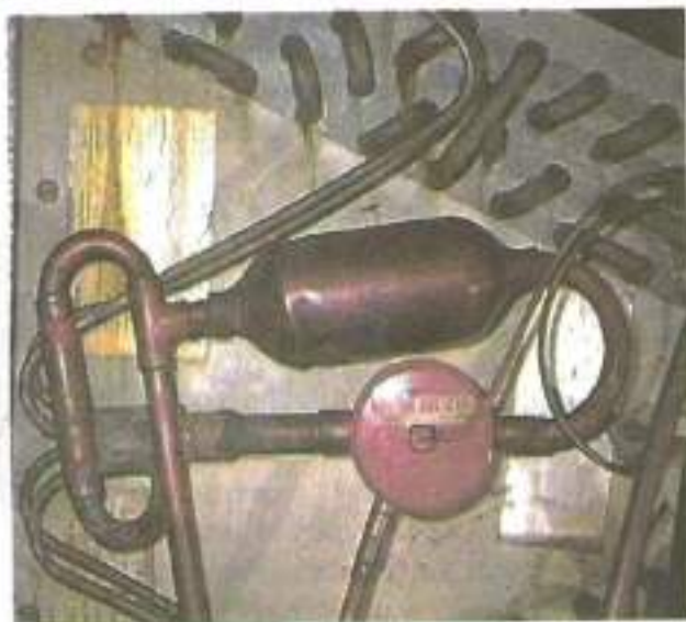
Thermostatic expansion valve.
