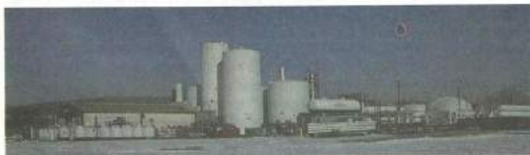
Manufacture of Hydrocarbon refrigerants.
